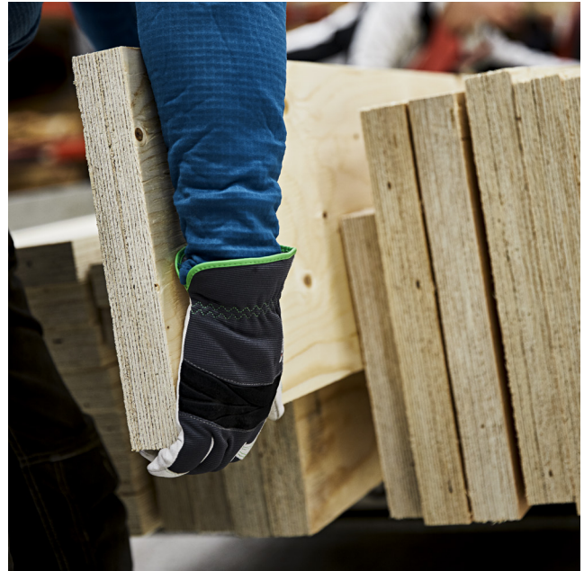
Figure 3.5. Handling of LVL beams
