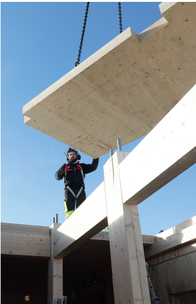
Figure 2.13. Installation of a multiple-glued GLVL-C floor element.
