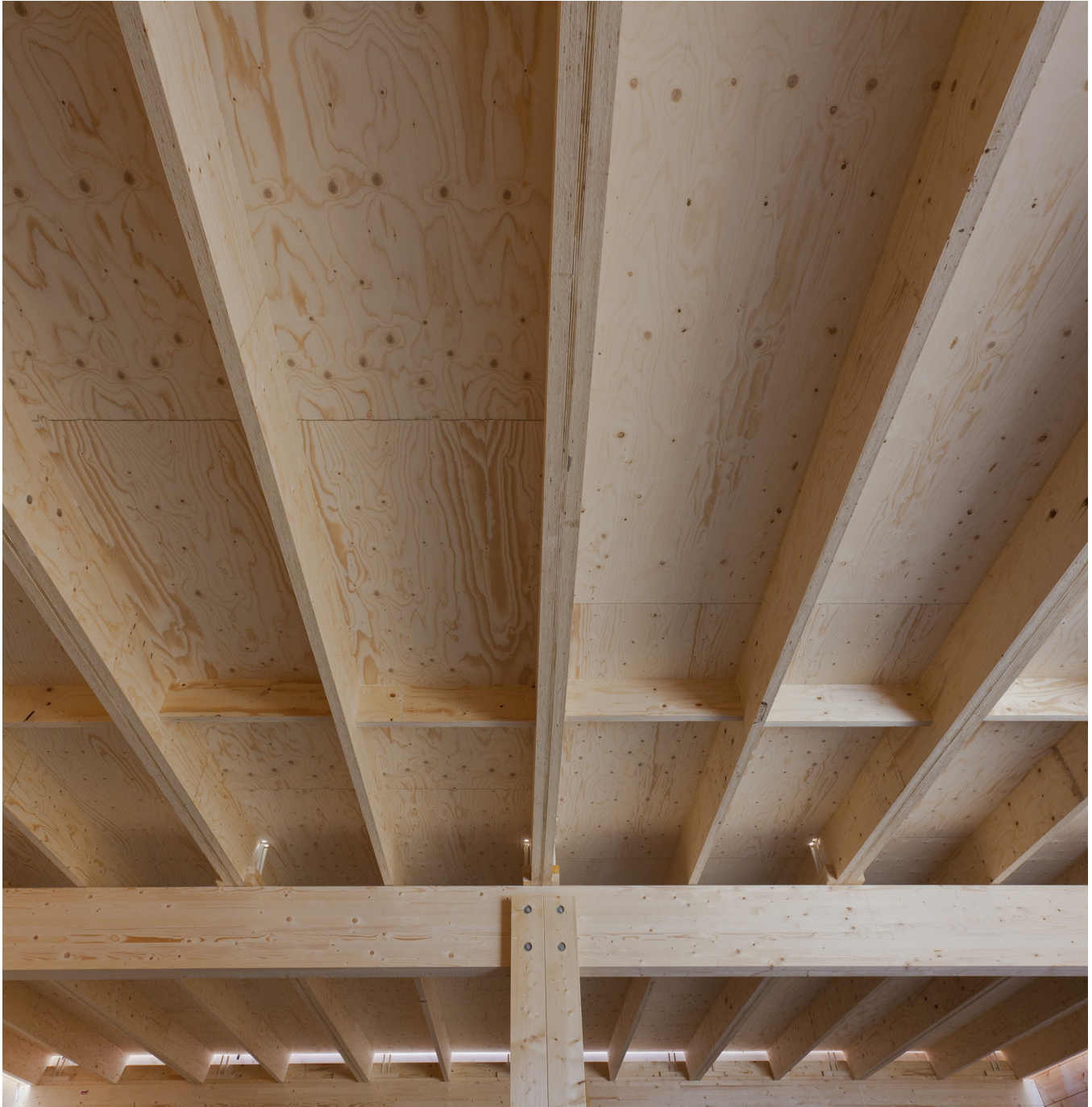
Figure 1.1 LVL roof structure, K-Rajamarket, Utsjoki, Finland.
