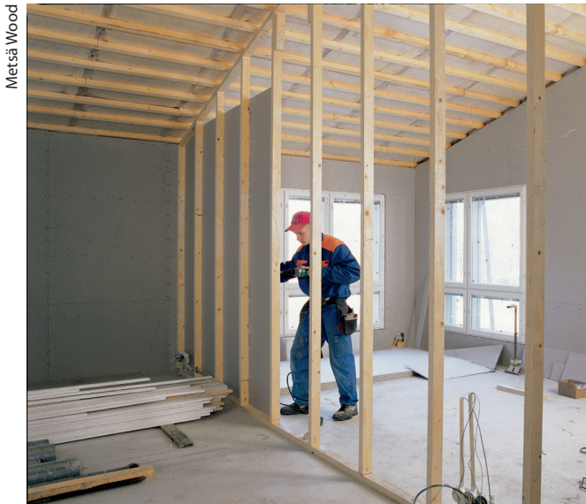
Figure 2.56. Installation of plasterboards to LVL-P wall studs.
