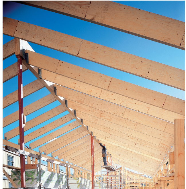
Figure 2.28. LVL-P rafters in a ridge roof structure.
