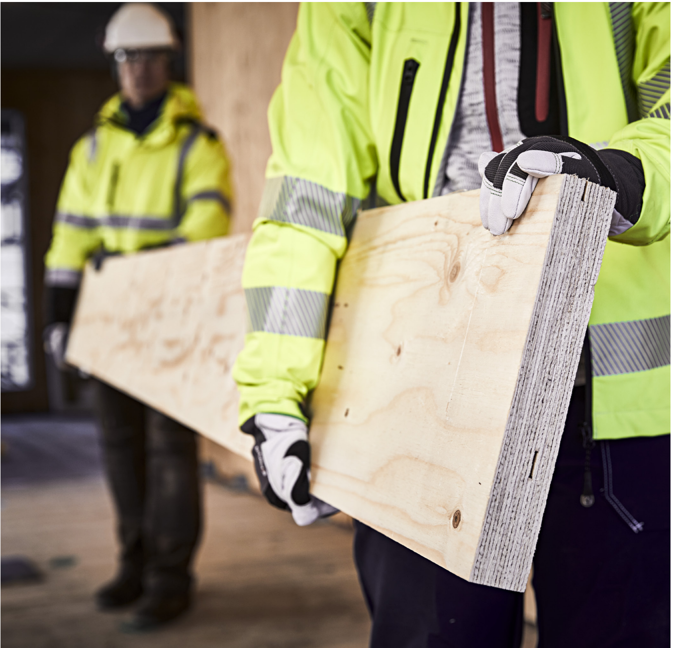
Figure 3.1. Handling of LVL beams
