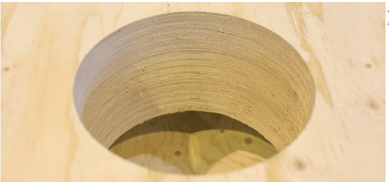
Figure 1.50. Hole in an LVL beam.
