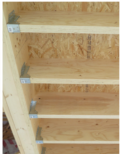
Figure 2.3. Joist hanger connections of floor joists.
