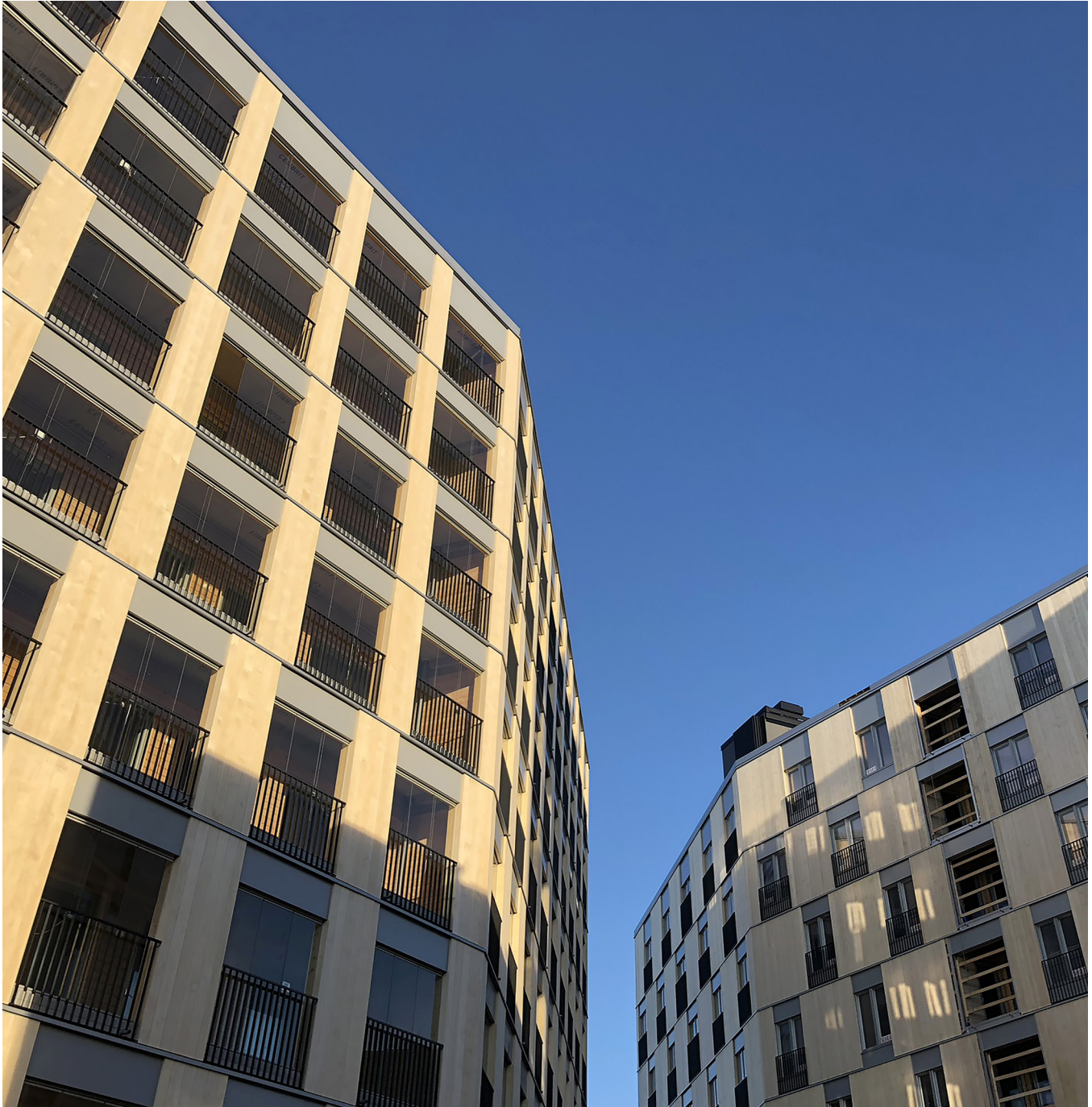
Figure 1.1 Wooden multi-storey building, Wood City, Helsinki, Finland.
