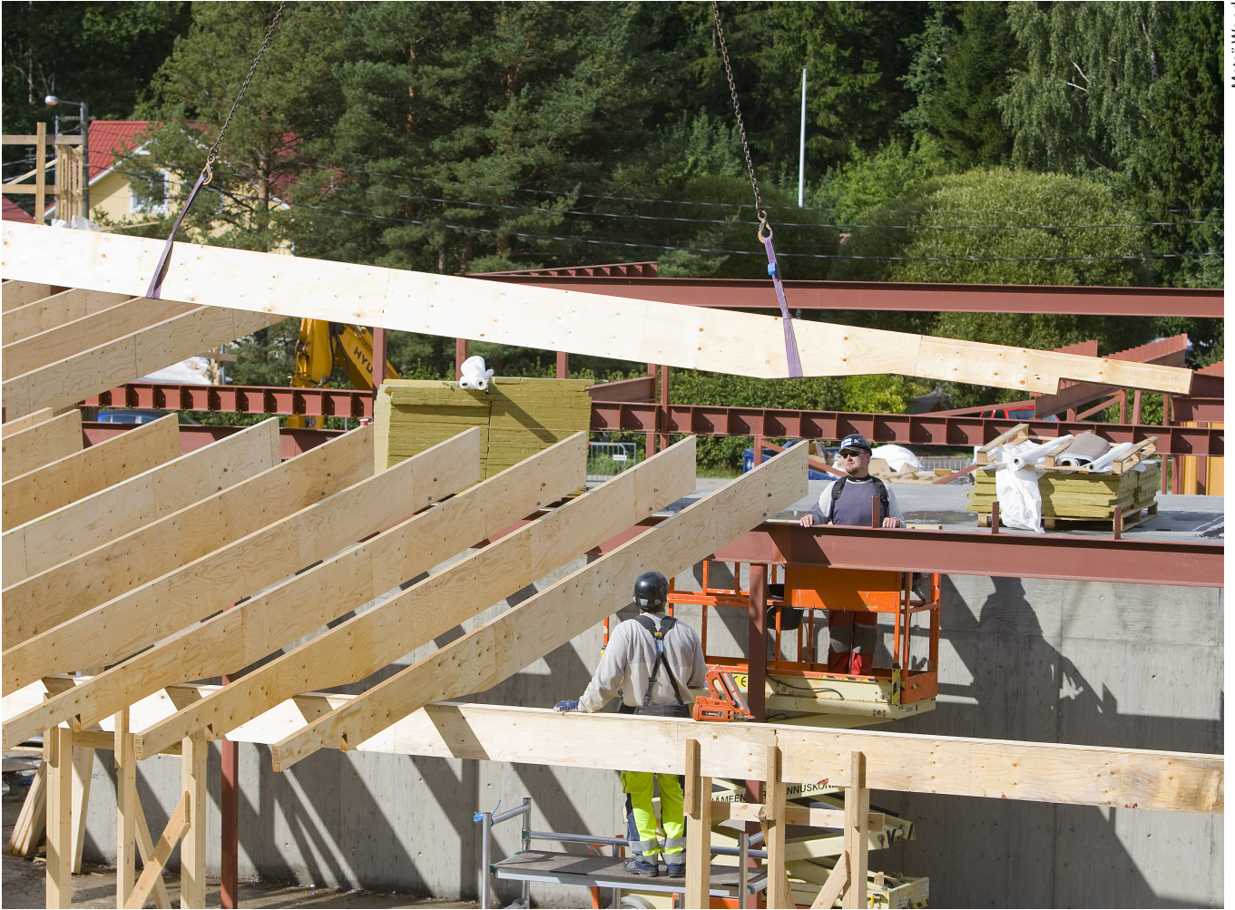
Figure 1.49. LVL-P roof beam cut to special shape.
