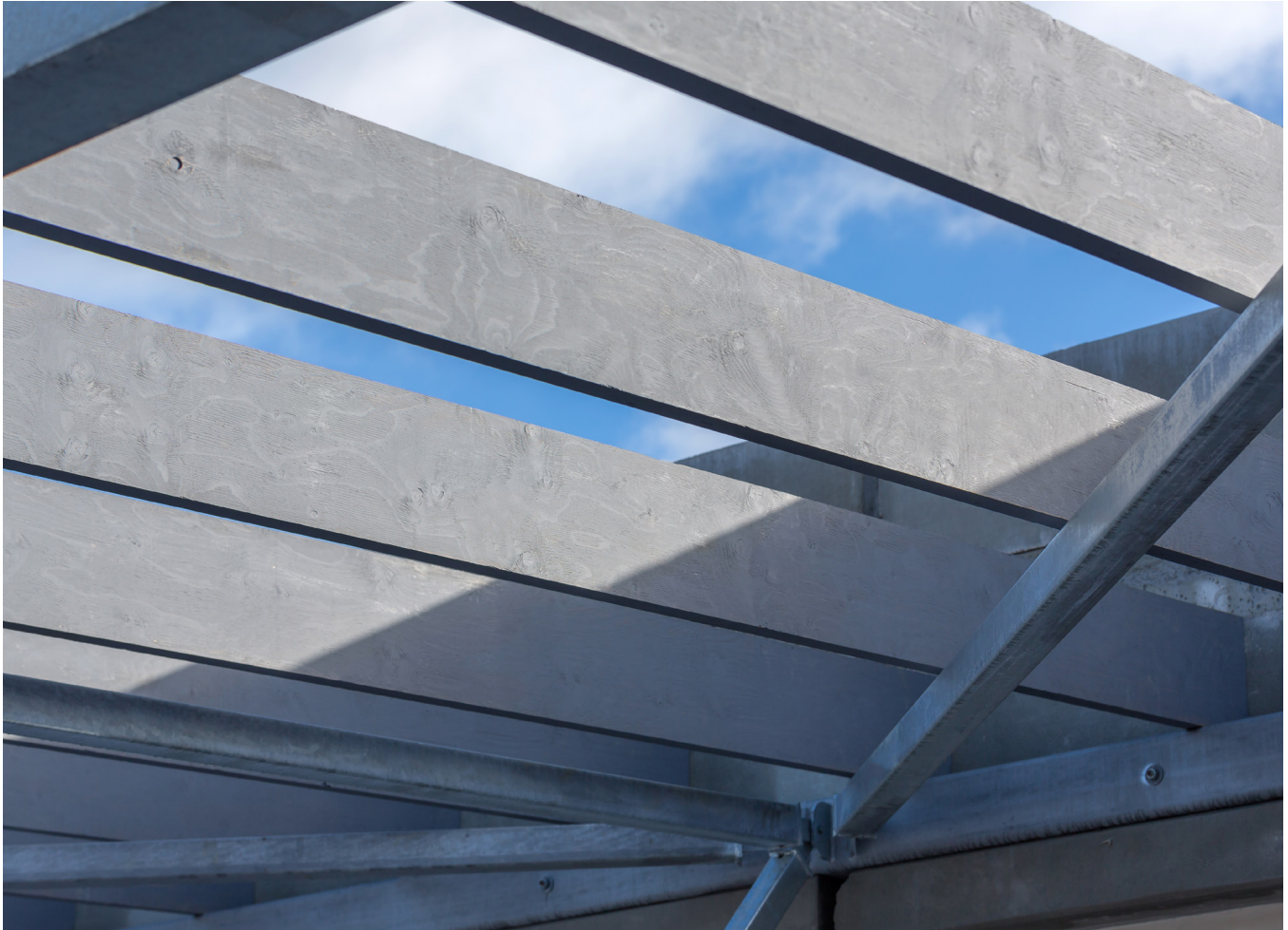
Figure 1.66. Coated surfaces of LVL beams.
