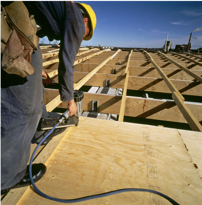
Figure 2.45. Installation of LVL-C roof panels.
