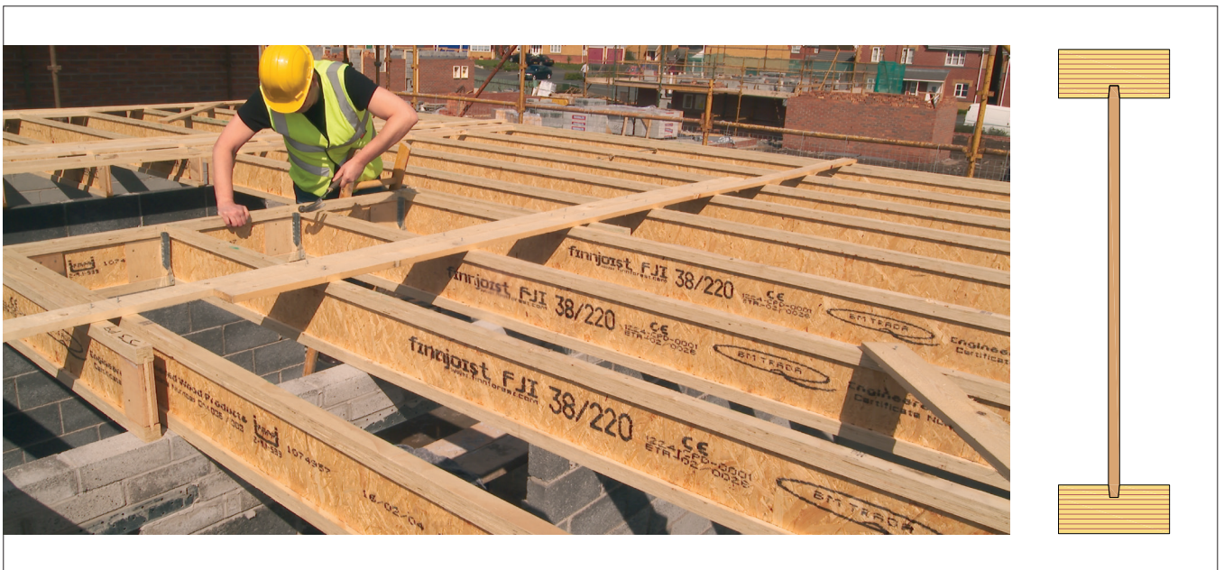
Figure 2.94. Wooden I-joist with LVL flanges.
