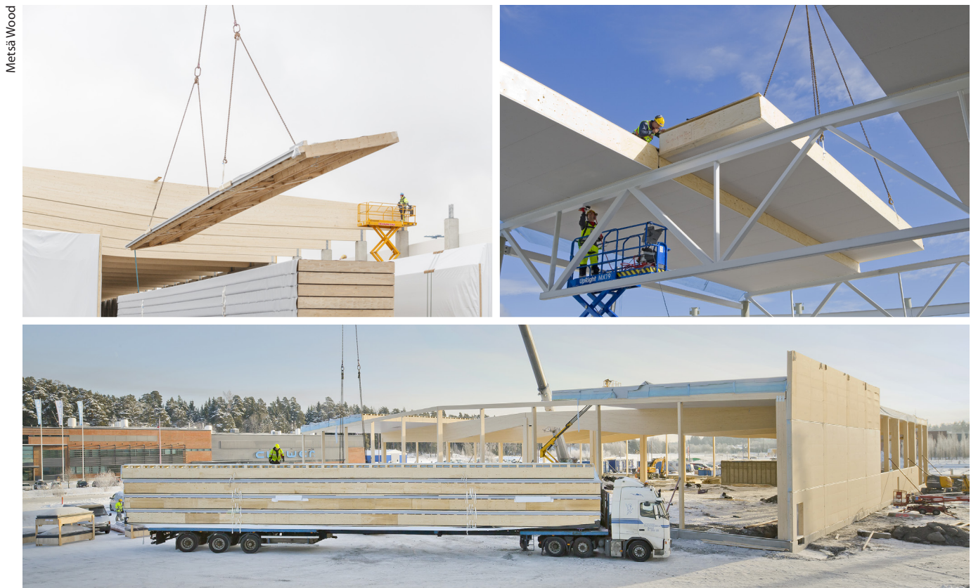
Figure 2.40. Installation of roof elements with LVL purlins. Metsä Fibre pulp terminal, Vuosaari, Helsinki, Finland; Karisma, Lahti, Finland; Skanssi, Turku, Finland.
