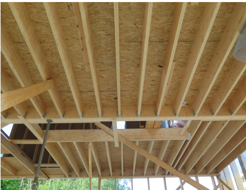
Figure 2.2. LVL-P joist floor structures.
