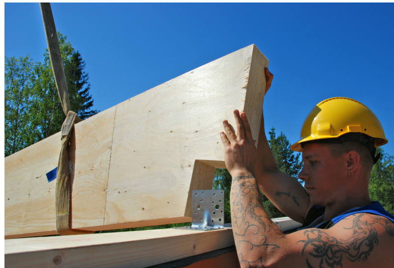
Figure 4.19. Installation of notched rafter beam.
