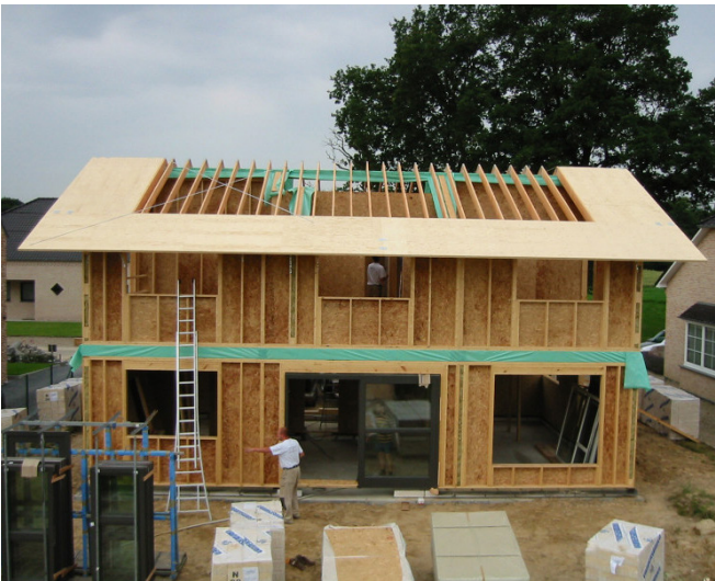
Figure 2.47. Eaves and roof overhangs from LVL-C panels.
