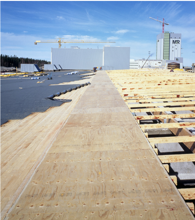
Figure 1.4 LVL-C roof panels.
