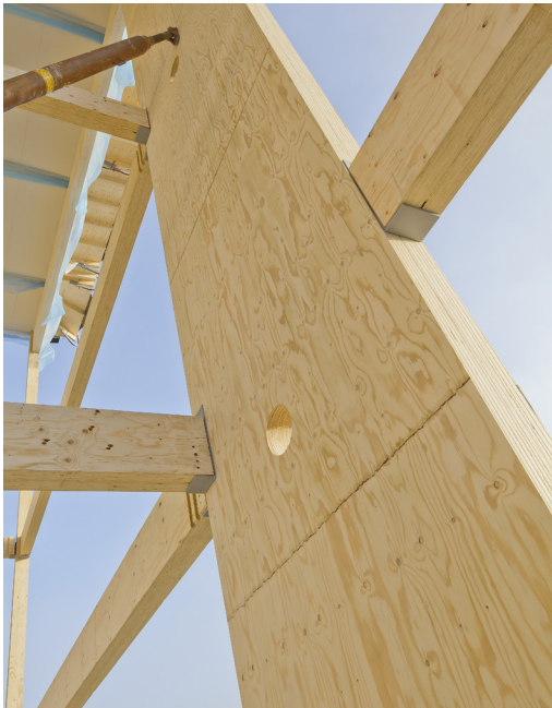
Figure 2.71. Multiple-glued GLVL-C bracing column.
