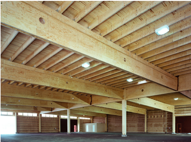
Figure 2.54. Large LVL I-beams as main beams of a warehouse roof structure at Herttoniemi, Helsinki, Finland.
