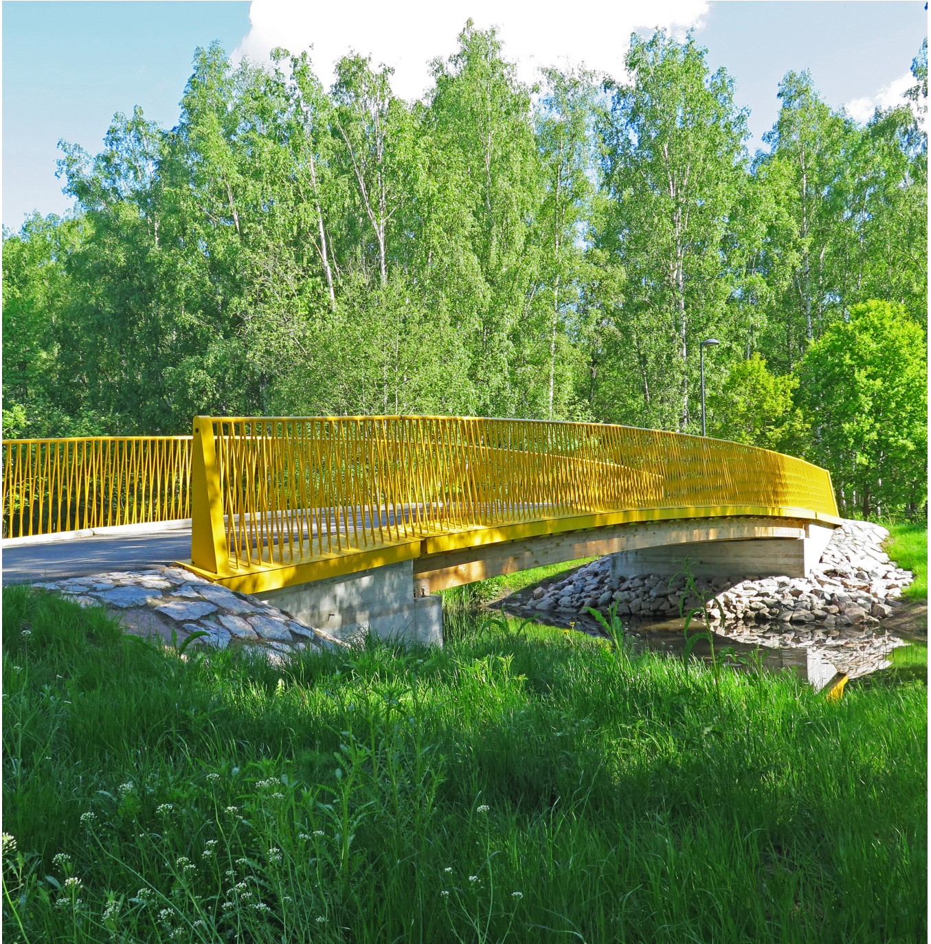
Figure 7.1. Wooden pedestrian bridge, Matinpuron, Espoo, Finland.
