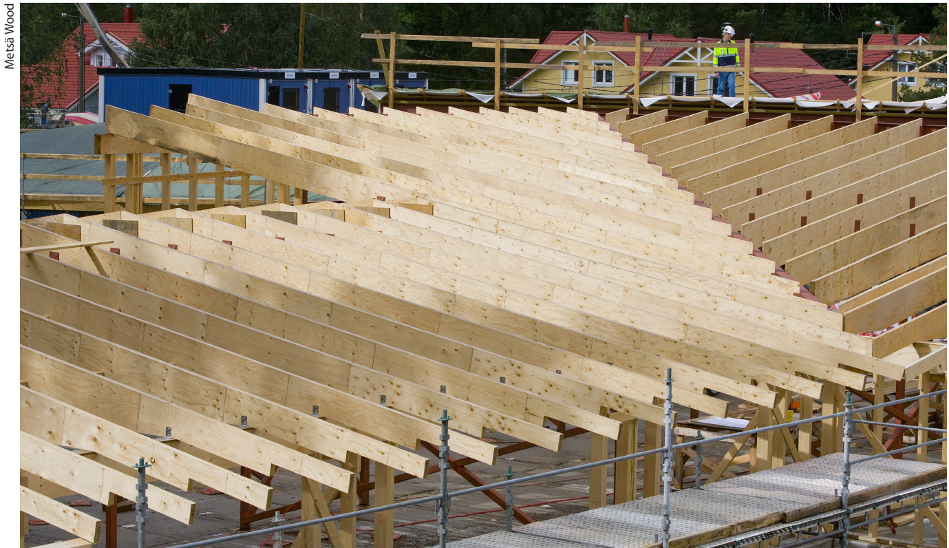
Figure 2.27. LVL-P rafters in a mono-pitch roof structure.
