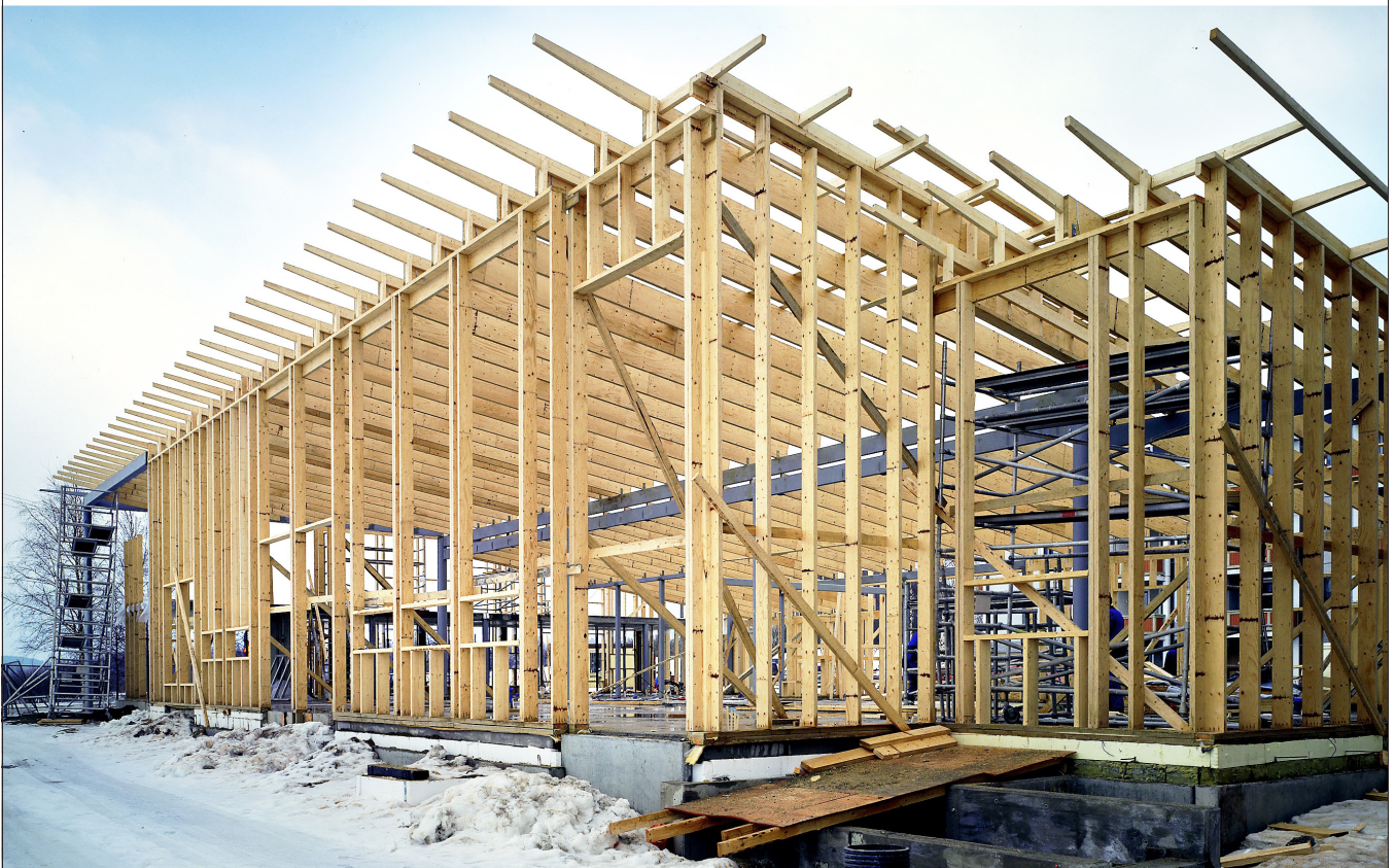
Figure 2.58. LVL-P studs for tall load-bearing exterior walls.
