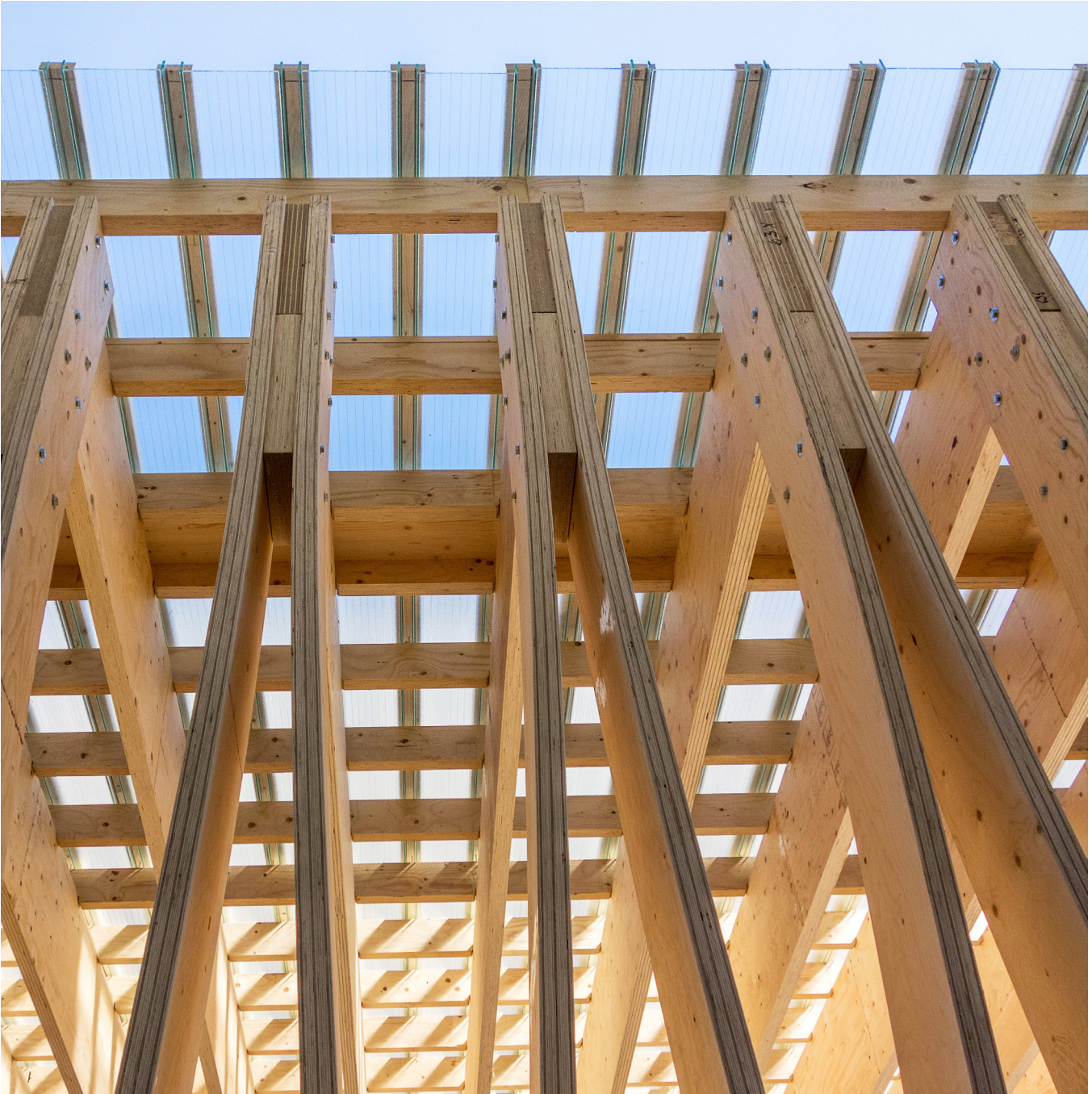
Figure 5.1. LVL connections.
