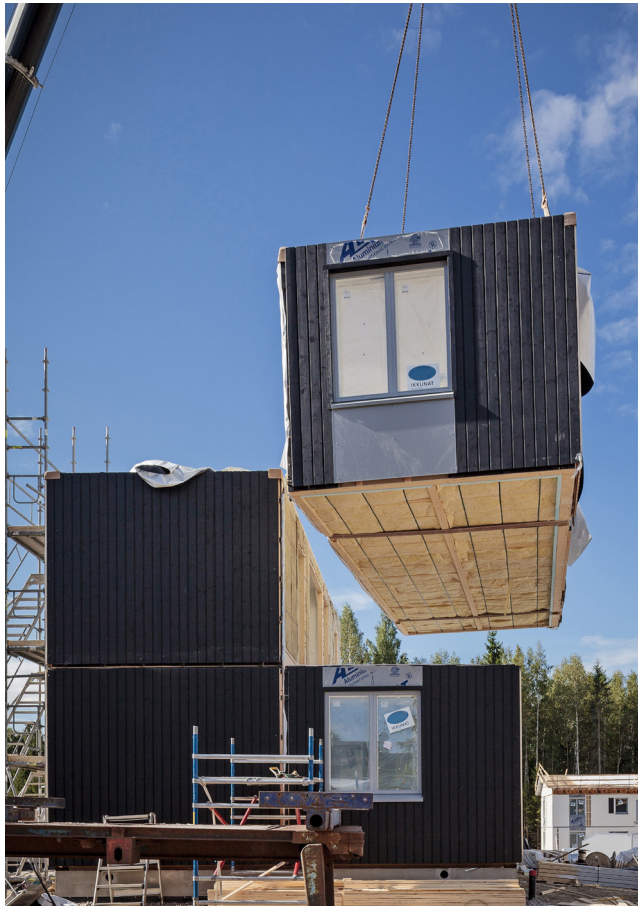
Figure 1.11 Off-site produced wooden volumetric elements, BoKloK, Vantaa, Finland.
