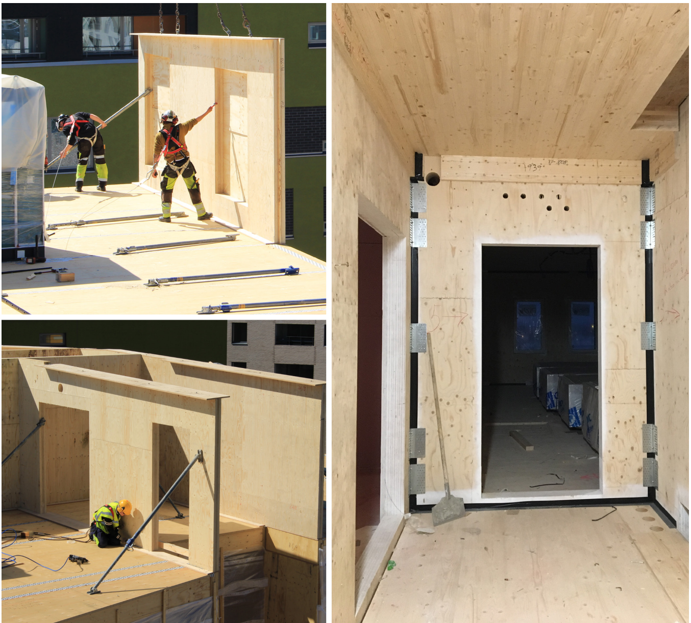
Figure 2.75. Multiple-glued GLVL-C panel walls.
